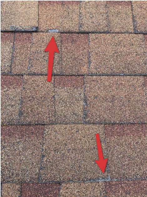
Damaged/torn shingles
