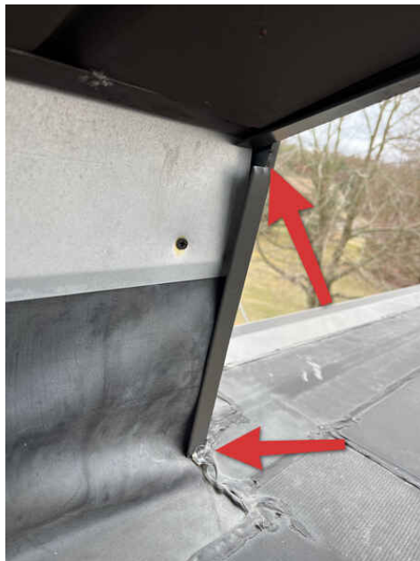
Failing sealant
