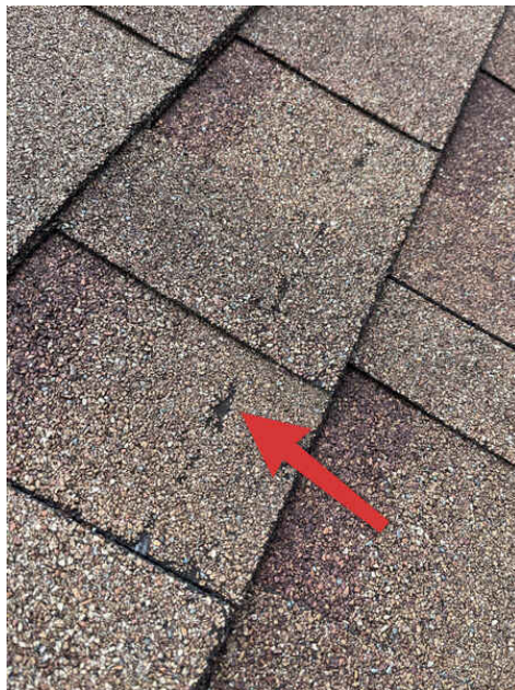
Damaged shingles
