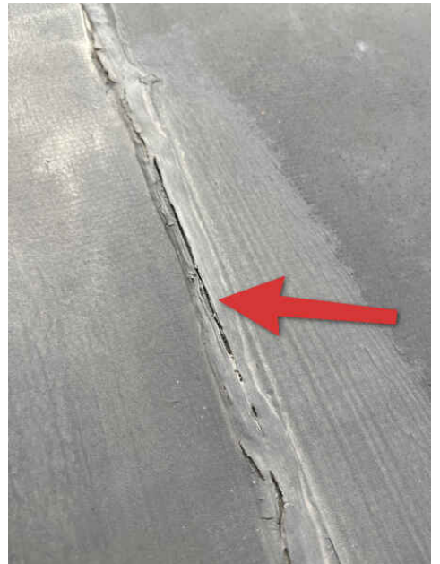
Failing sealant
