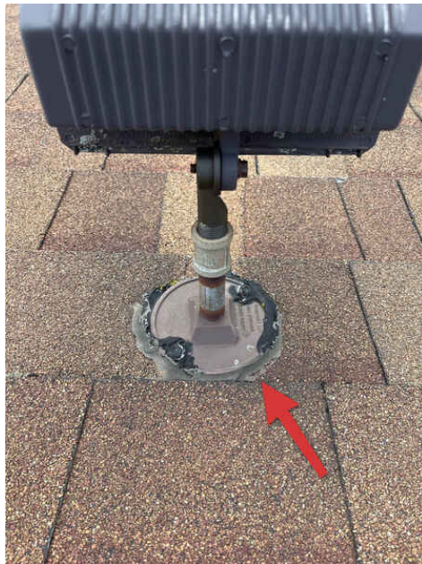
Failing sealant
