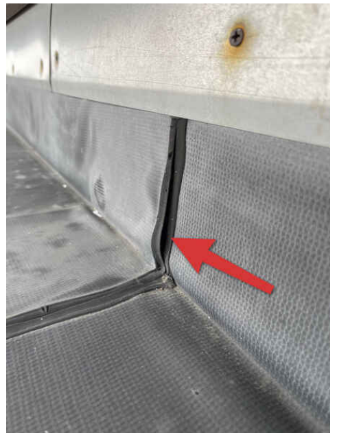
Failing sealant
