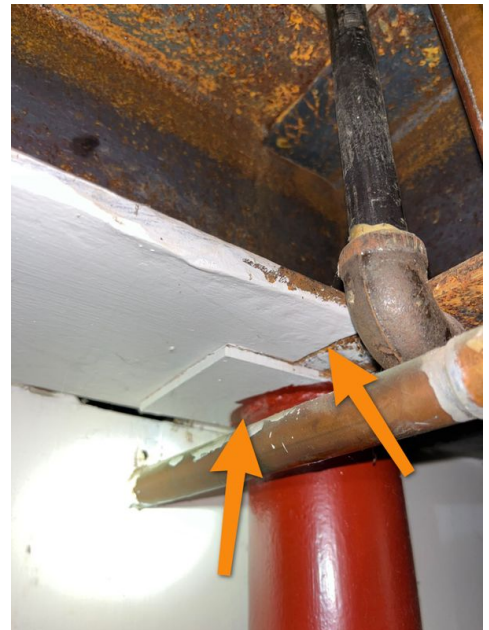
Near basement staircase
