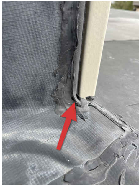
Failing sealant
