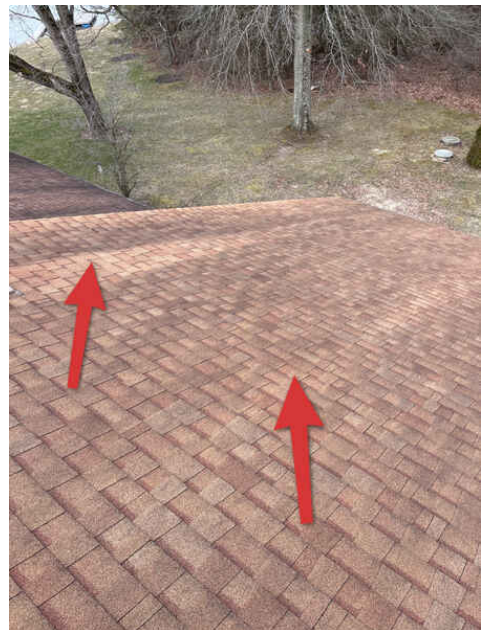
Moderate granule loss
