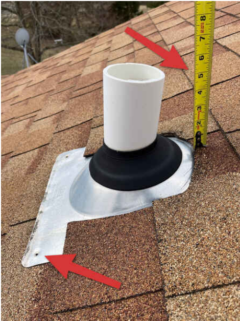
Missing fasteners and plumbing vent improper height
