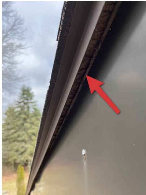
Missing flashing
