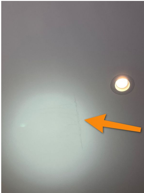
Living Room Ceiling
