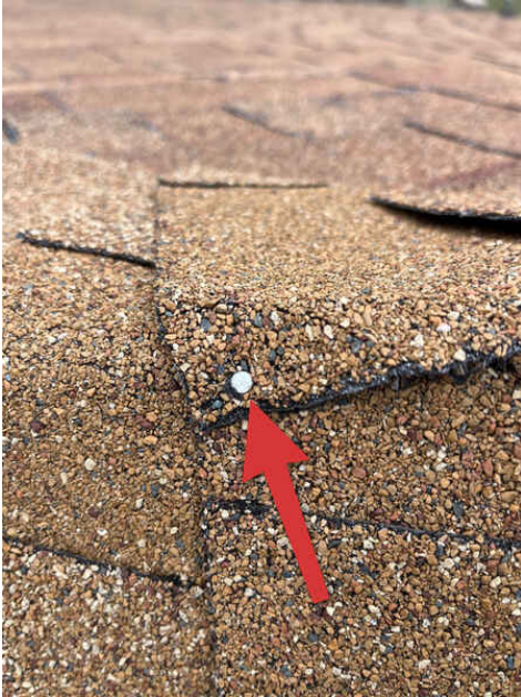
Exposed fasteners
