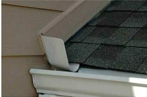
Here is an image of proper kick-out flashing from a different home.
