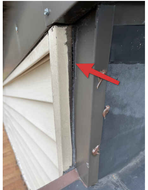
Failing sealant
