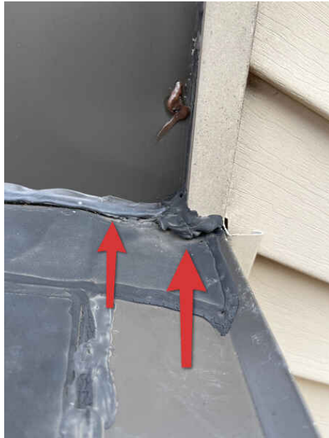
Failing sealant
