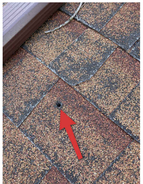
Damaged shingles
