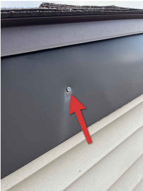
Exposed fasteners
